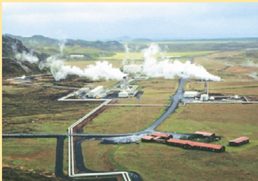
Geothermal power plant in Iceland
